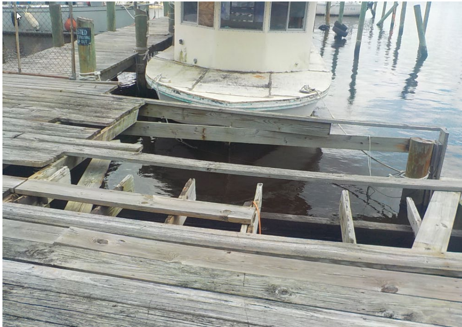
Figure 3: View of dilapidated dock.
