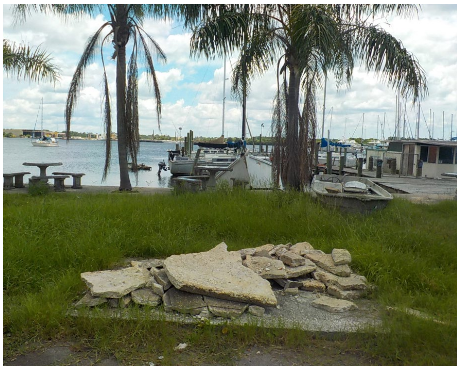
Figure 1: General view of facility.
